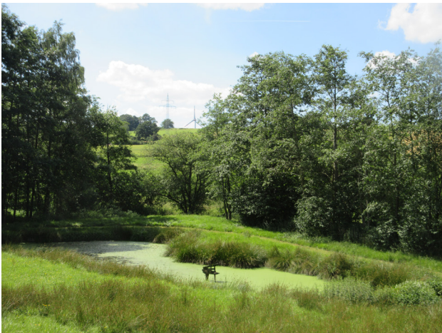
Photo 5 The maturation pond of the pond sewage plant in Dirlammen with algae growing during July. Photo credit: C. Opp 2017
