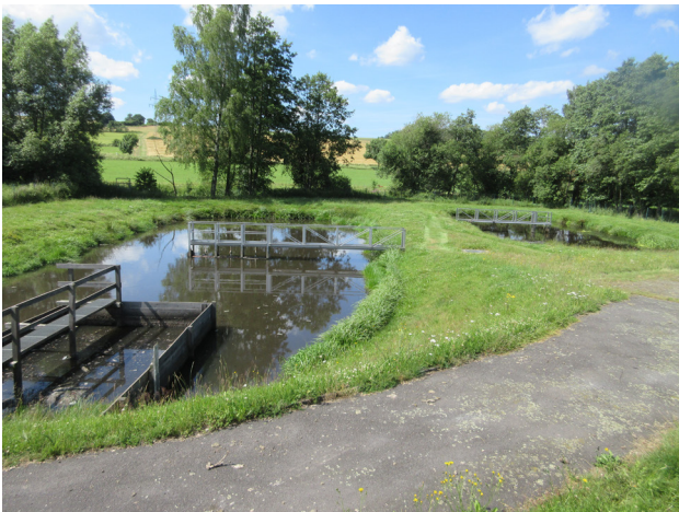
Photo 4 First and second air conditioned pond of the pond sewage plant in Dirlammen. Photo credit: C. Opp 2017
